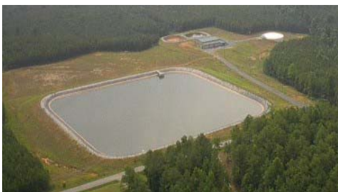
Snake Creek Water Plant Complex
