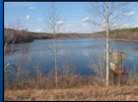
Existing NRCS Dam
