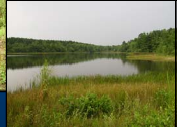
Existing NRCS Dam
